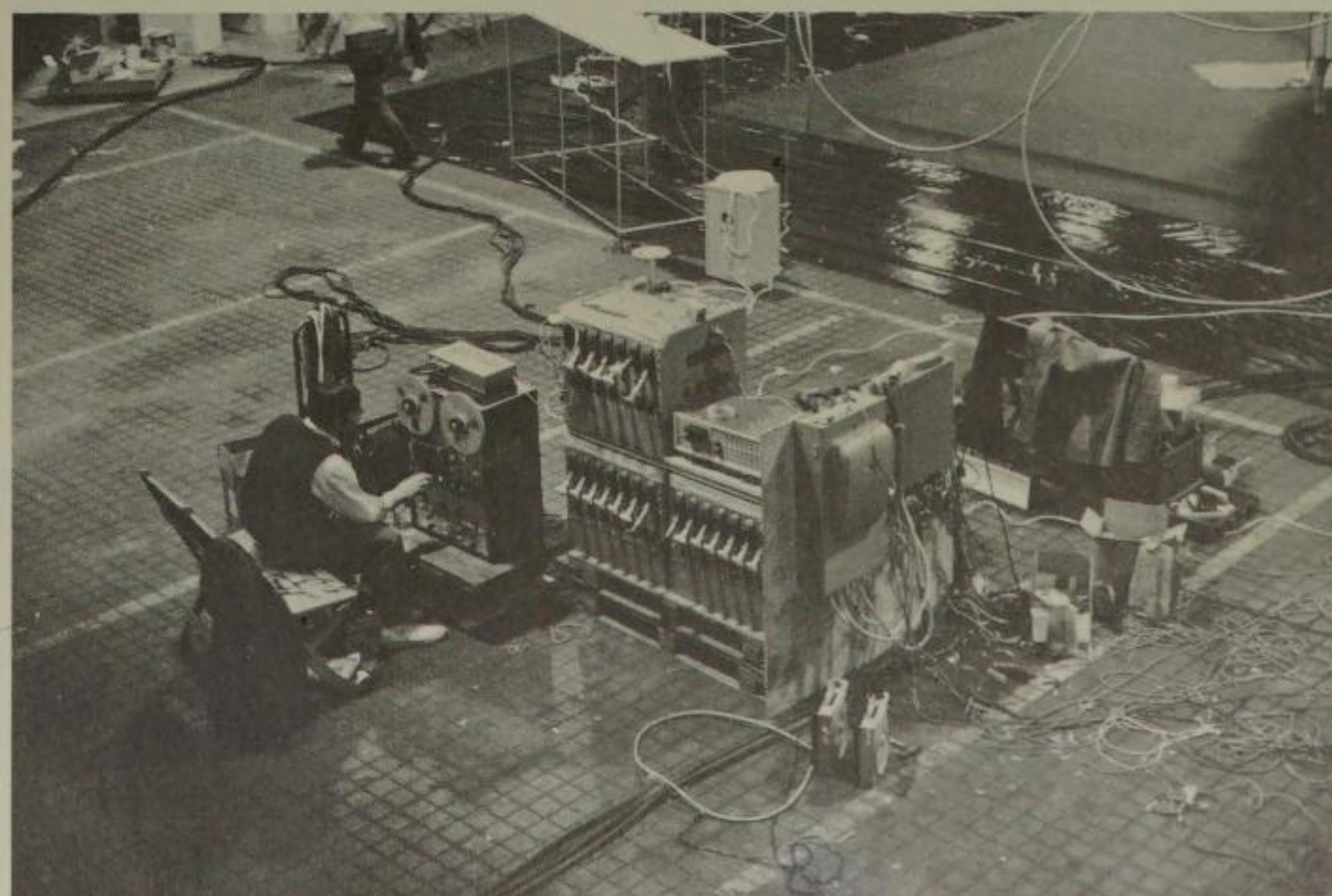
9-69. Control center outside the dome, including computer, quadrasonic tape deck, and lighting controls.
