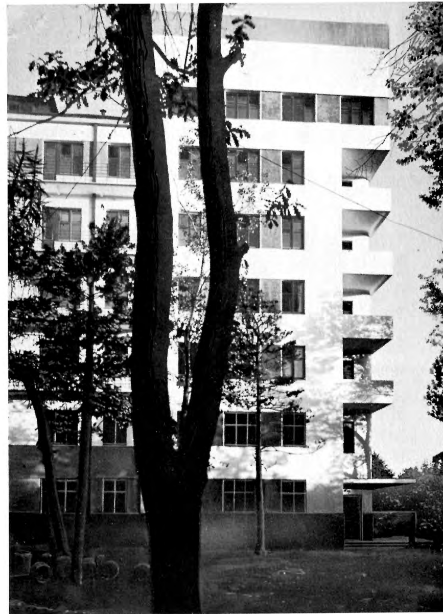
Plate 16. Apartment building constructed by Mossoviet.
