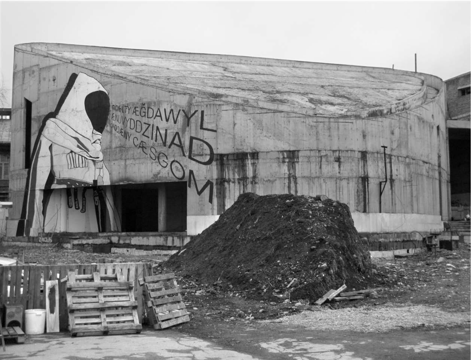
Museum under construction, Vladikavkaz, North Ossetia
