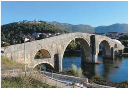
Arslanagić Bridge, Trebinje
