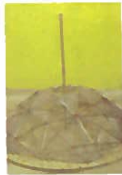
Construction of the dome from top to bottom, assembly mast, around 1948
