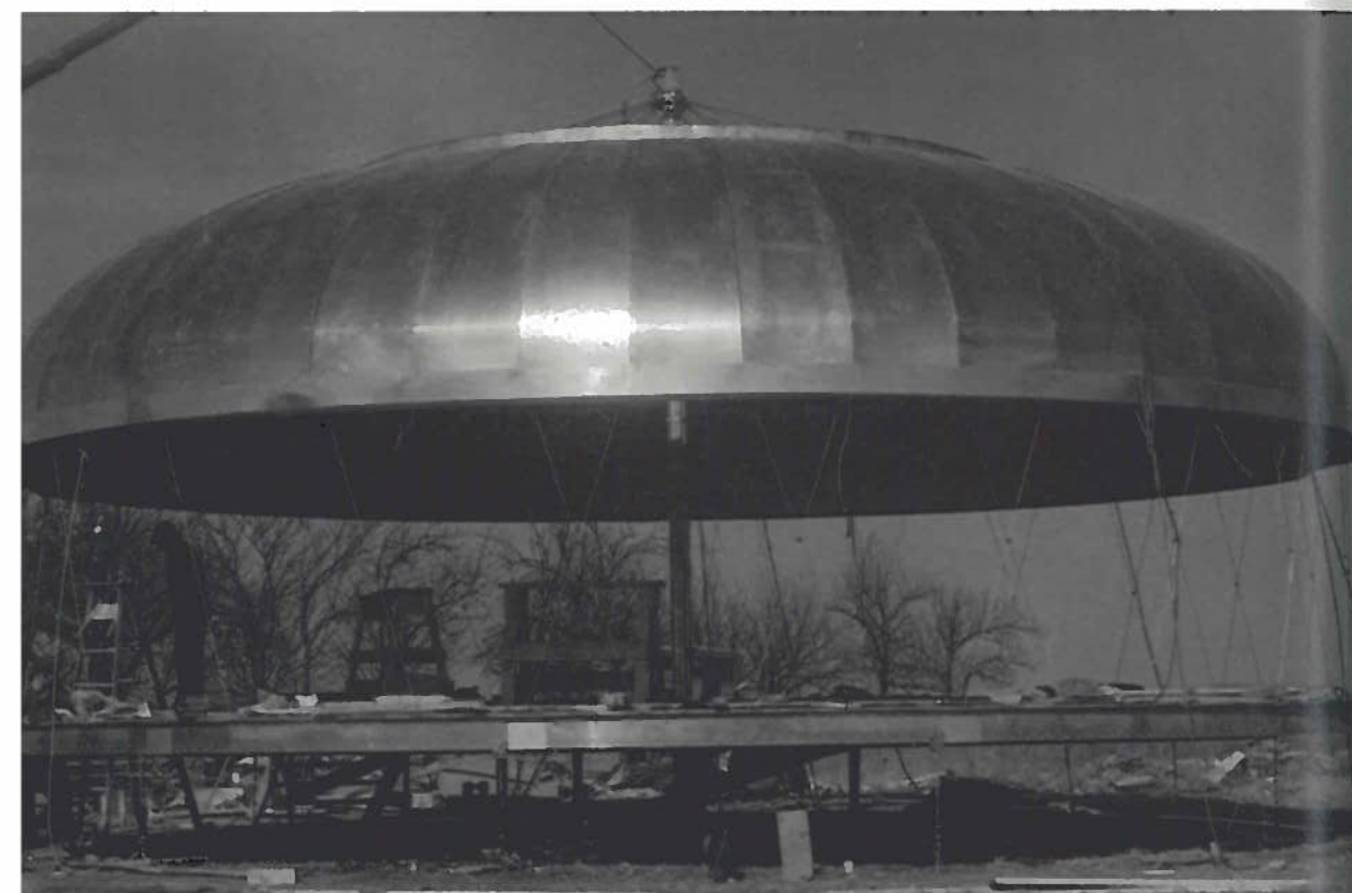
844 The dome is hoisted up on the mast.
