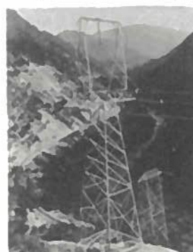
10 Snow type dead end suspension tower
