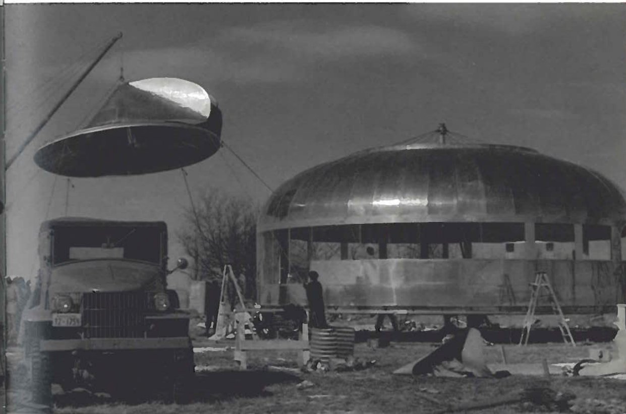
845 The ventilator is pulled in place. Parapet and windows have been assembled.
