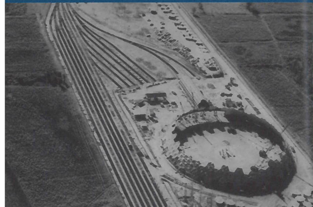
330 - Dome for the Union Tank Car Company, Baton Rouge; aerial photograph after the beginning of construction (Fall 1958) and photograph of the finished dome (October 1958)
