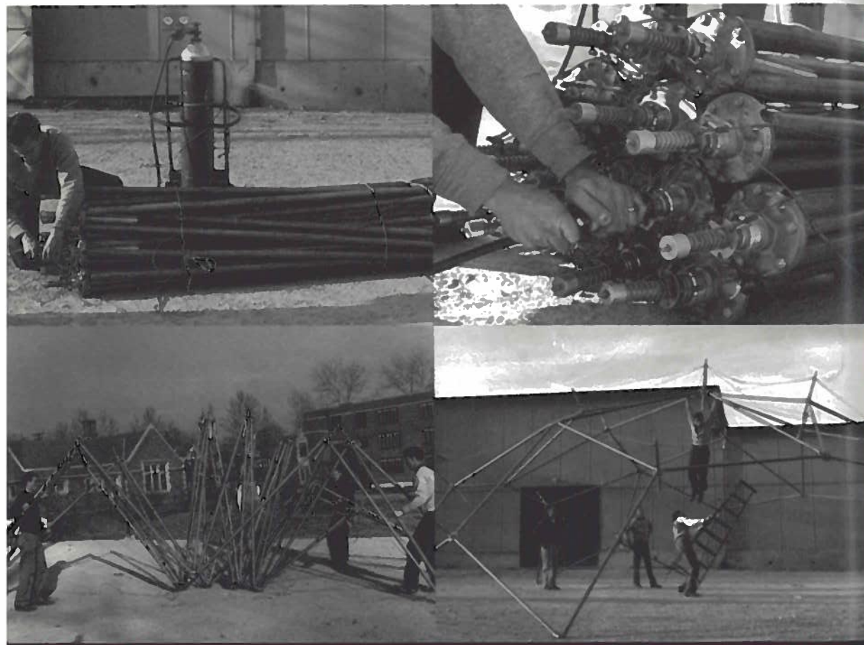
848 - Flying Seedpod: project at Washington University, St. Louis, 1953; geodesic structure able to fold up, developed with an eye toward later use in space travel
