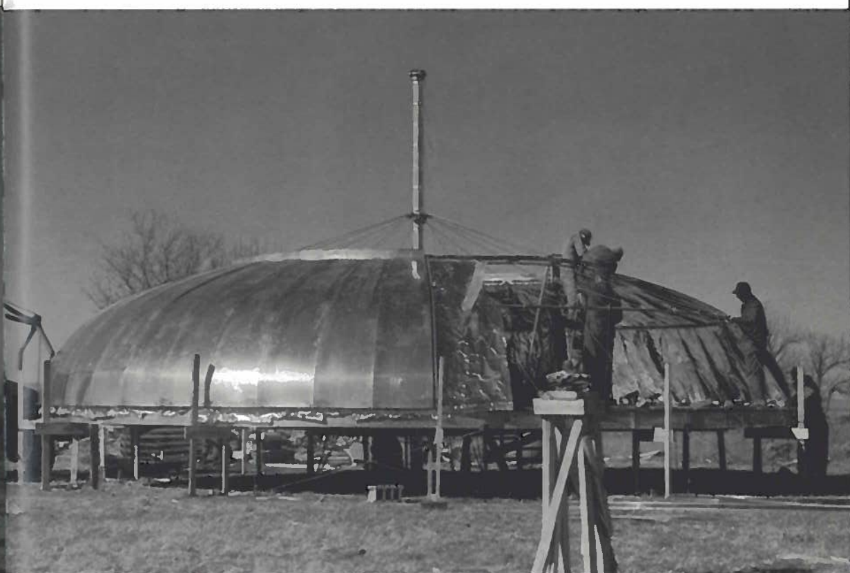
241 Cladding the structure with thermal felt on the inside; aluminum sheeting on the outside.
