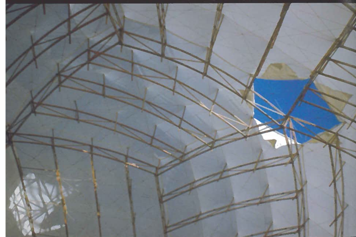
332 Dome in Aspen, wooden slats and outer plastic skin, 1958
