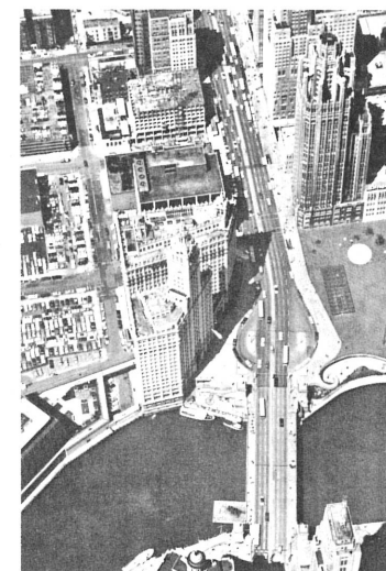
Michigan Avenue Bridge Looking North Chicago, Illinois
