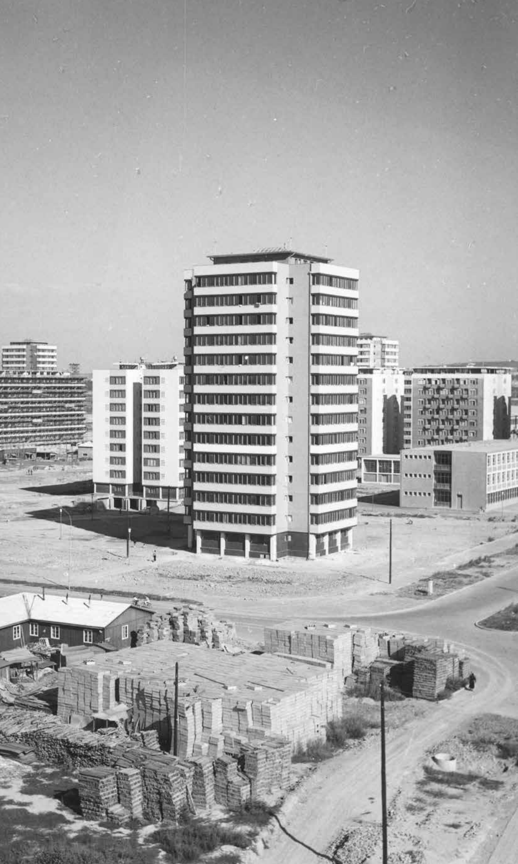
Construction of the first blocks in New Belgrade, Milan Pavlović, Source: Historical Archives of Belgrade, Ur_11979
